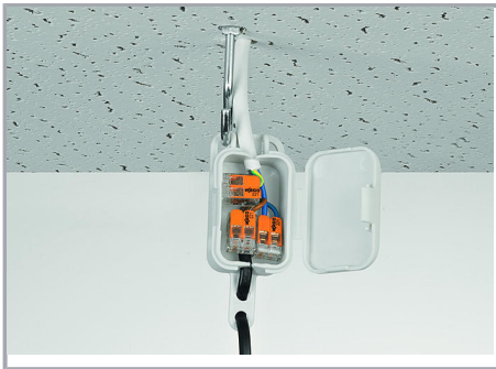
Pendant light connection in a suspended ceiling
